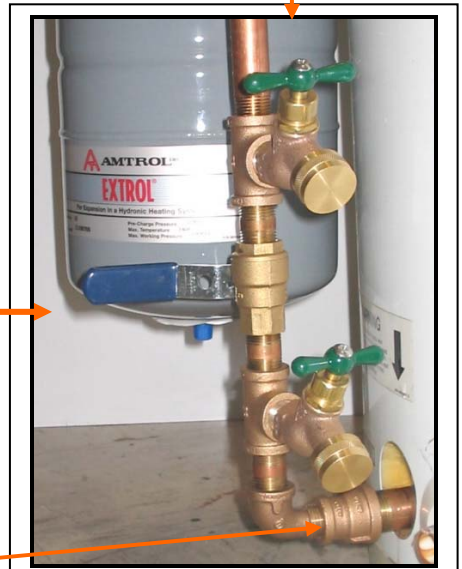
Charging Valve Assembly
