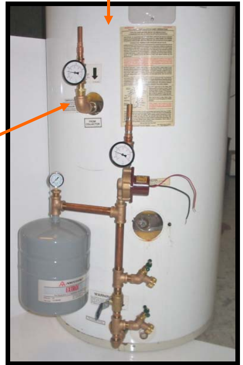
Charging Valve Assembly
