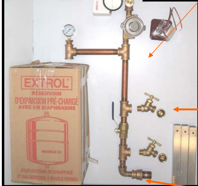
Charging Valve Assembly
