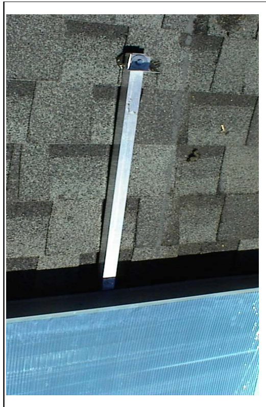
Above: Top EII Bracket in place and ready for top collector to be installed.
