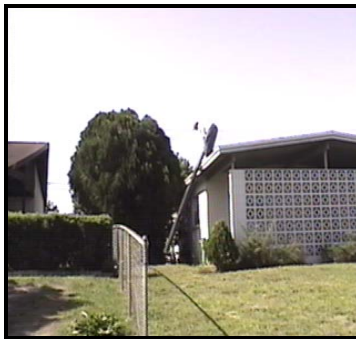
Keeping your body weight over the Roof, pull the Collector Up
